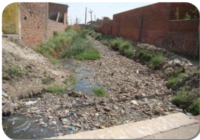
Pic 7: Drain in Panipat. 12.4.10
